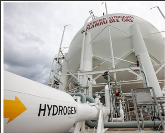
Figure 4: 20 m diameter LH 2 storage tank in NASA Kennedy Space Centre, Courtesy of NASA
